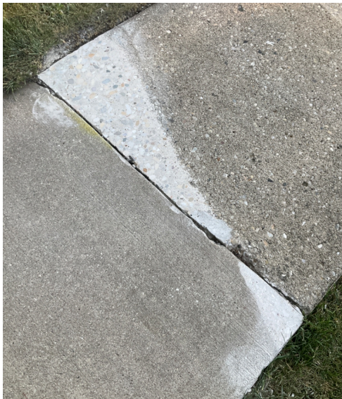
Sample Repair Photo: Defect 2 repaired on 09/10/2025 at 701 Sweetbriar PI at 5:52 PM
